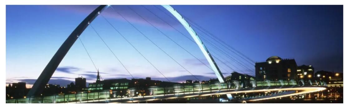
The surface of the arch is cross lit with simple elegant white light, although we also included the option of changing coloured light for special events. The underside of the bridge deck is lit with narrow beam sources directed along the structural ribs and the belly of the pedestrian deck, maximising potential reflections in the river surface.
